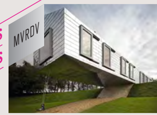
BALANCING BARN Suffolk, England
